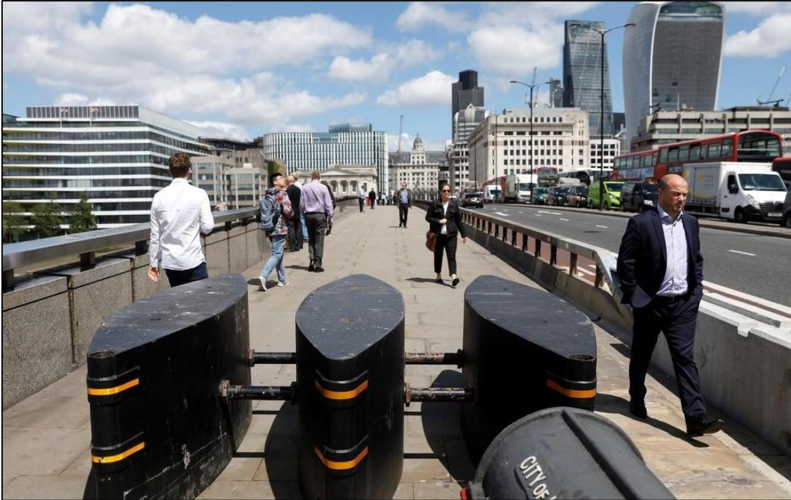
Plate 3 - Vehicle Security Barriers (VSBs) preventing vehicular access to footway on London Bridge. Note that these VSBs are mounted on the bridge deck itself, and the size and weight of these units is a direct result of the lack of depth available for foundation.
