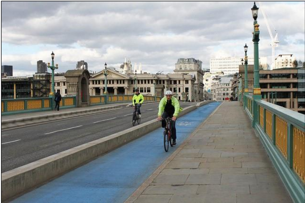
Plate 5 - Revised HVM barriers between cycle track and general traffic lanes on Southwark Bridge
