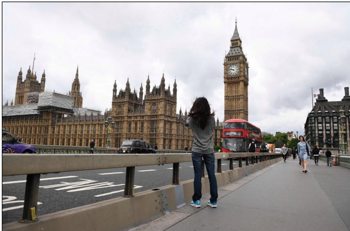
Plate 2 - Kerbside location of Varioguard type barriers on Westminster Bridge
